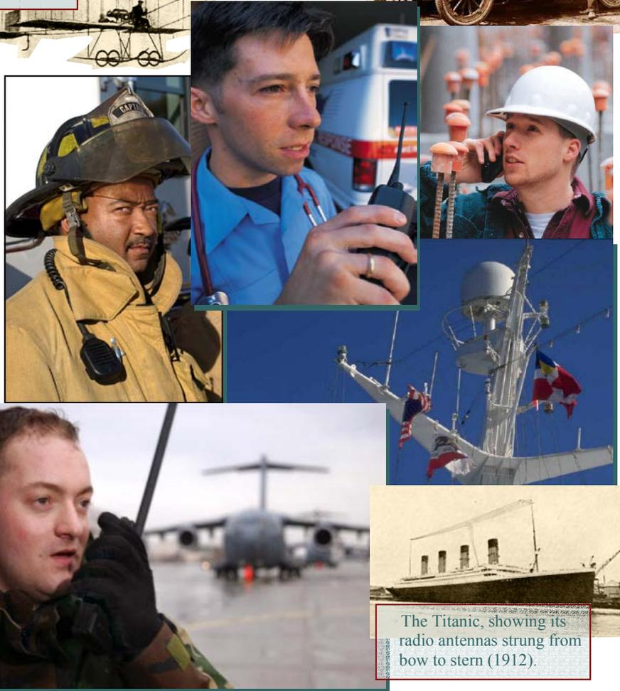
The Titanic, showing its radio antennas strung from bow to stern (1912).
